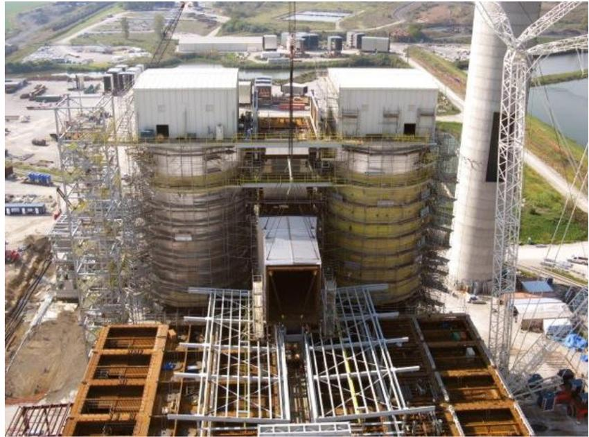
Boilermakers from Local 363 are installing a scrubber system at Dynegey’s Baldwin Energy Complex in Baldwin, Illinois
