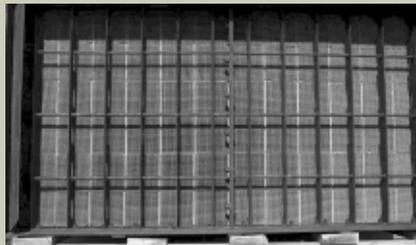
**6. Cleaned catalyst.** The cleaned catalyst modules from Plant Gorgas were returned to the SCR system for reinstallation and operation. Meanwhile, a full layer of catalyst from Plant Bowen's Unit 1 was cleaned and stored for future use. *Courtesy: Southern Company*
