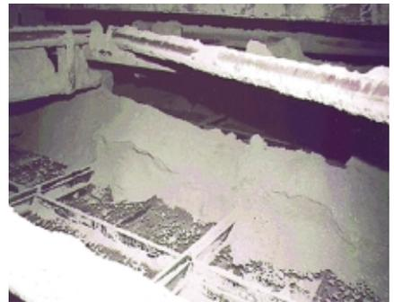
**3. SCR reactor with heavy ash.** This picture shows a German SCR with heavy ash buildup from close spacing of catalyst levels and equipment located too near the catalyst face. *Courtesy: Argillon LLC*
