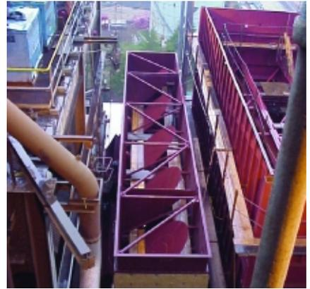
**2. Mix it up.** The Delta Wing being installed here on a new SCR uses large, angled disks to stimulate the mixing of NO<sub>x</sub>, ammonia, and temperature throughout the SCR inlet duct. *Courtesy: Babcock Power Environmental Inc.*
